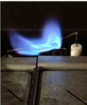
Normal Pilot Flame Pattern
