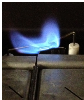
Normal Pilot Flame Pattern
