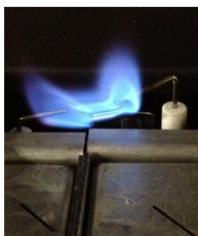
Normal Pilot Flame Pattern
