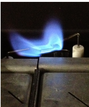
Normal Pilot Flame Pattern
