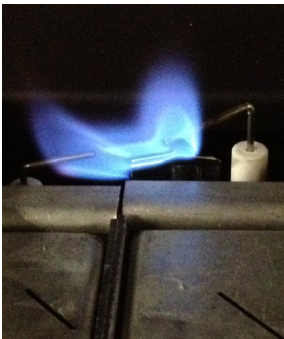
Normal Pilot Flame Pattern
